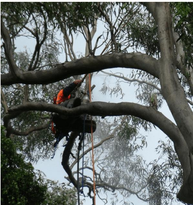
Figure 25. Sprinklers being installed in trees by Sunshine Coast Council
