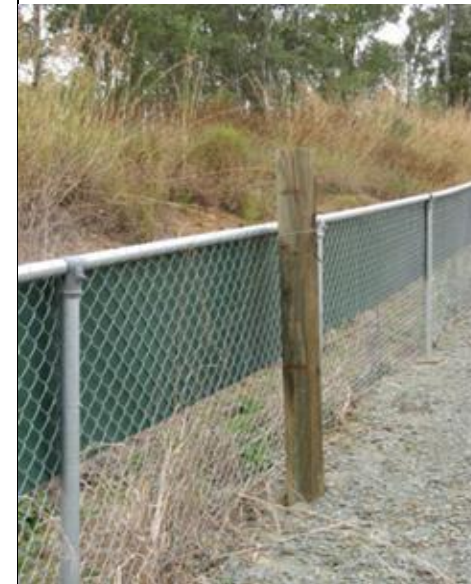
Figure 4.3.22. (photo D de Villiers) Escape poles placed along a road corridor will allow koalas to exit the road corridor and jump over the koala exclusion fencing to the safety of adjacent habitat.
