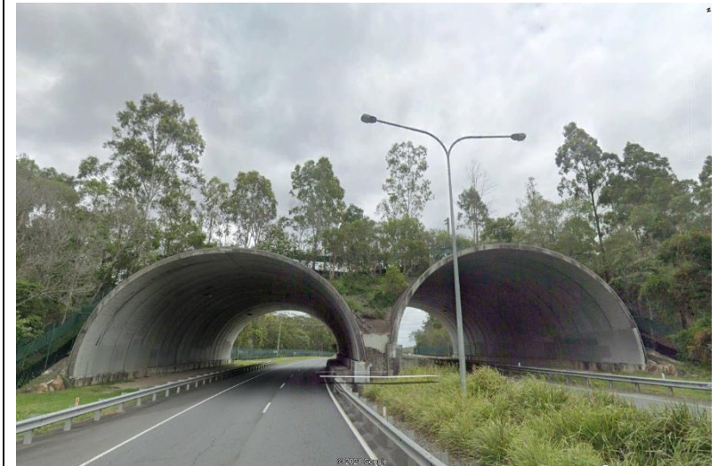
Figure 4.3.9. (photo: google earth) A landbridge designed for use by wildlife has well established trees and ground cover to facilitate crossing.
