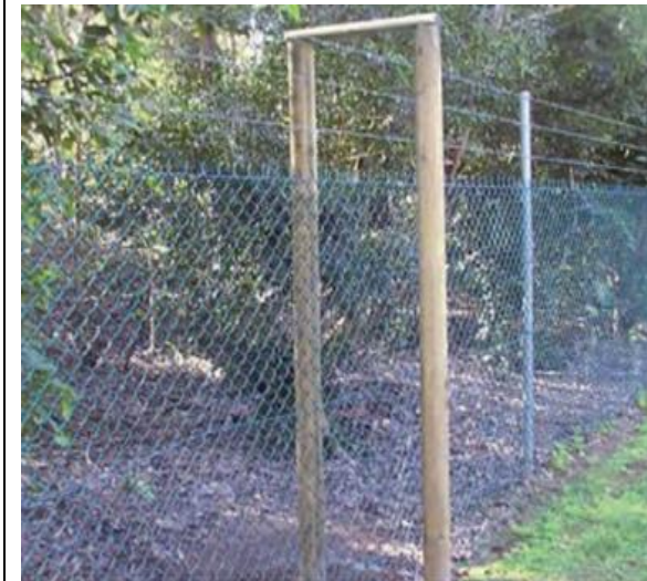
Figure 4.1.4. A wooden bridge over security fencing designed to facilitate the safe movement over the fence and barbed wire by koalas but effectiveness is not well established.
