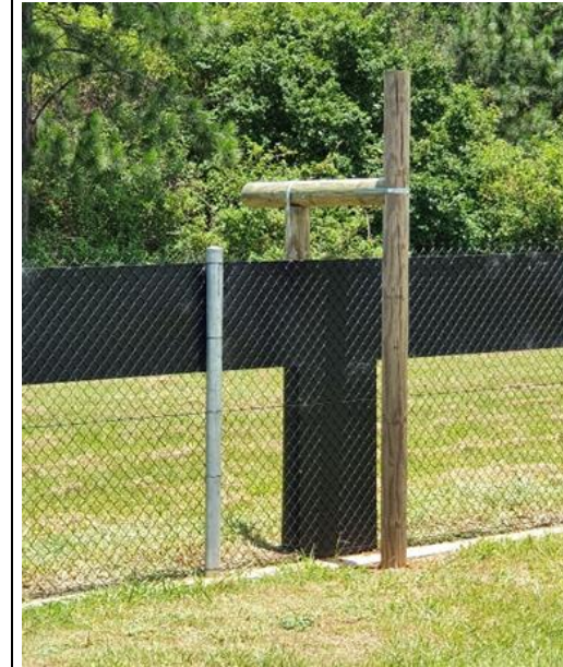
Figure 4.3.19. (photo D de Villiers) A double-sided escape pole may facilitate the more rapid exit of koalas from a transport corridor. Metal sheeting on the habitat side stops koalas from climbing the fence and reaching the pole above the sheeting.
