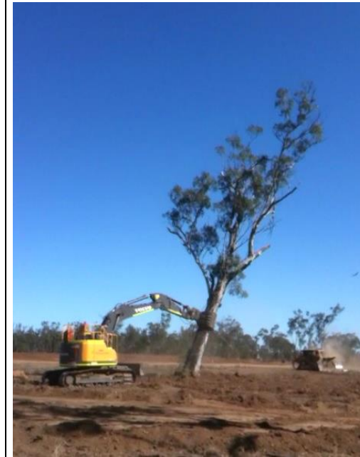
Figure 4.4.5.(photo: Brian Coulter ) An excavator with a tree grab can gently lower trees to the ground, reducing the risk of broad-scale clearing and felling on fauna such as the koala.
