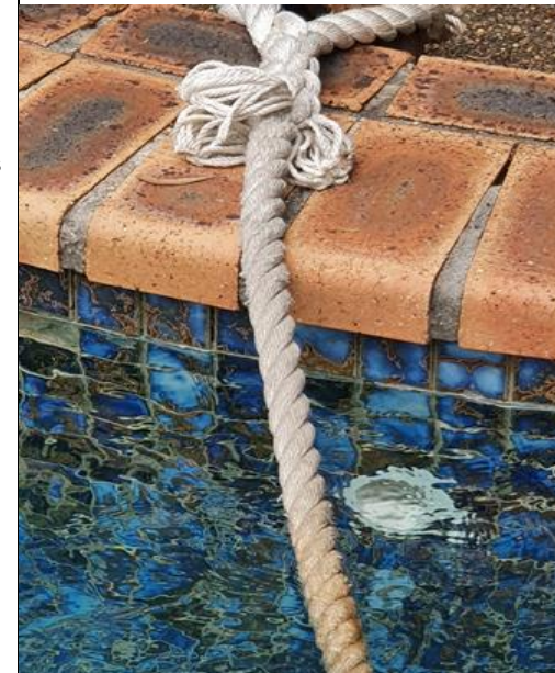
Figure 4.6.3. (photo: D de Villiers) Large diameter marine rope securely anchored to a structure beyond the pool can provide a point of egress out of the water and be placed at opposite ends of a pool.
