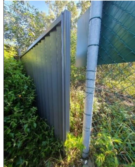
Figure 4.2.8. (photo D de Villiers) Reduced fencing height creates a partial barrier to koalas and discourages koalas climbing the fence and entering the road corridor.
