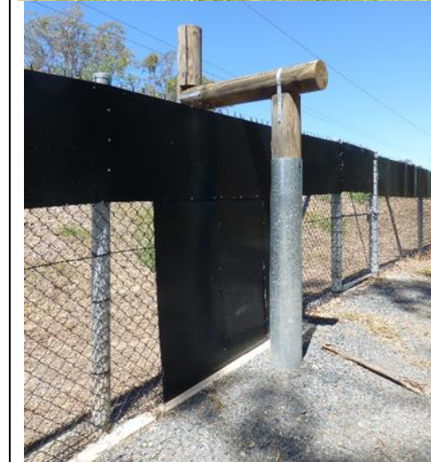
Figure 4.3.20. (photo D de Villiers) The ingress pole on the habitat side of the fence must prohibit climbing by koalas – here the pole is fitted with smooth metal sheeting and the fence adjacent to the pole is pannelled to stop koalas climbing the chain-link fencing and grabbing the pole above the metal collar.
