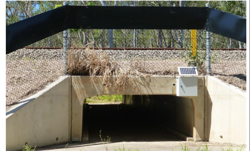
Figure 4.3.14. (photo D de Villiers) Small 900 mm box culverts can still provide movement opportunities for koalas but are too small for the installation of koala furniture and will have reduced natural light penetration.
