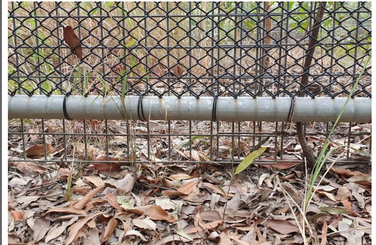
Figure 4.2.6. (photo D de Villiers) Fencing can be retrofitted with additional wire cover gaps under koala proof fencing where the ground is undulating.
