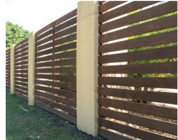
Figure 4.1.3. Small-spaced fencing slats allow koalas to climb the fence while reducing entrapment between slats.
