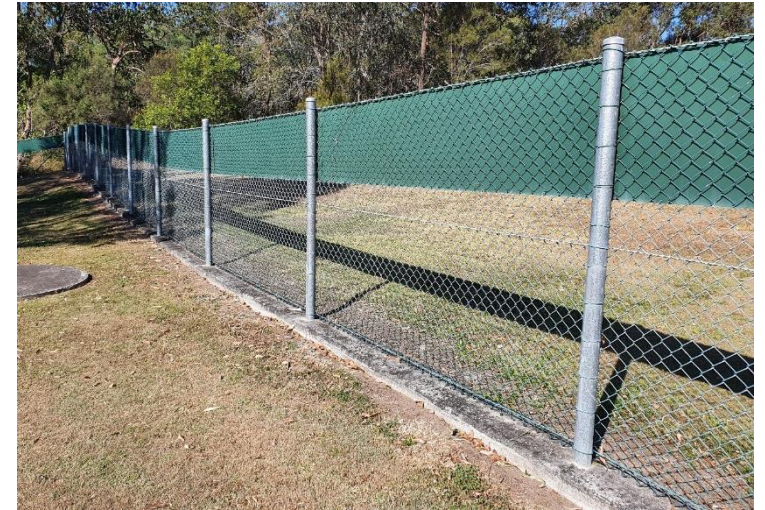
Figure 4.2.1. (photo D de Villiers) Koala exclusion fencing with unclimbable sheeting on the habitat side of the fence prevents koala access to the road corridor or other unsafe environments. Fencing is flush with a cement footing to prohibit koalas pushing under the fence.
