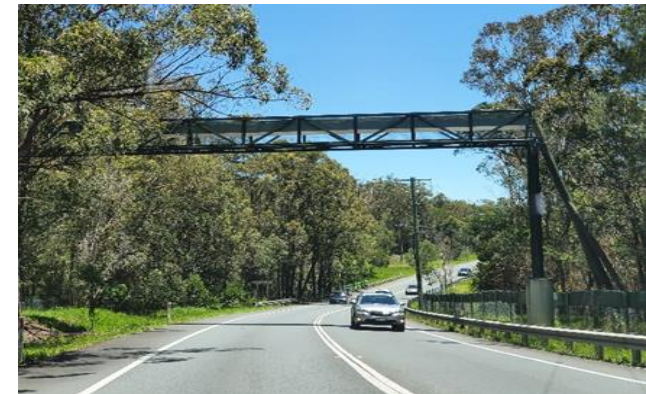
Figure 4.3.10. (photo: google earth). A fauna overpass links habitat on either side of a main road.
