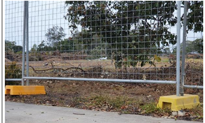
Figure 4.4.3.(photo D de Villiers) Temporary fencing is typically secured on footings with panels raised off the ground. This design allows egress of fauna into unsafe areas during clearing operations or in the construction zone.
